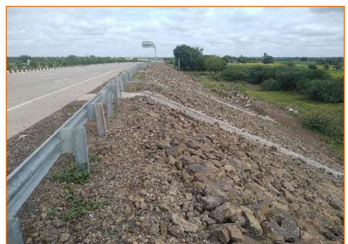
Slope Protection work at km. 298+300
