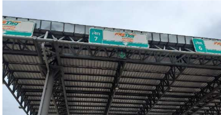
Figure 9-9 Over Head Lane Signal (OHLS)
