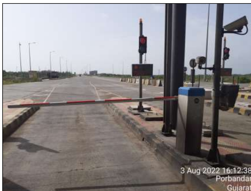
Figure 9-6 Automatic Lane Barrier
