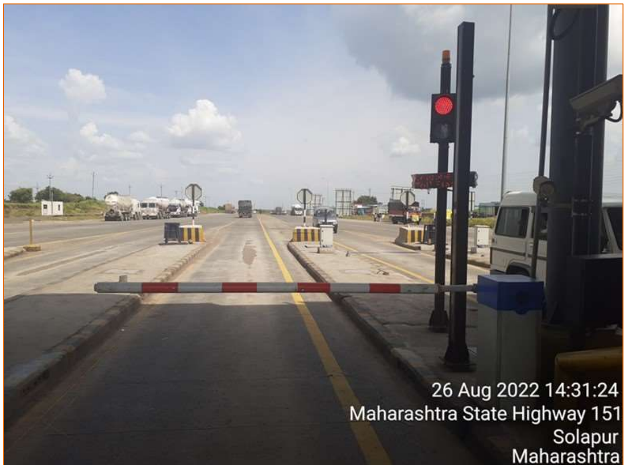
Figure 9-4 Automatic Lane Barrier
