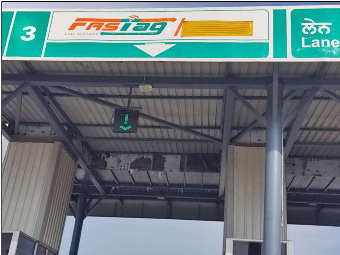
Figure 9-10 Over Head Lane Signal (OHLS)
