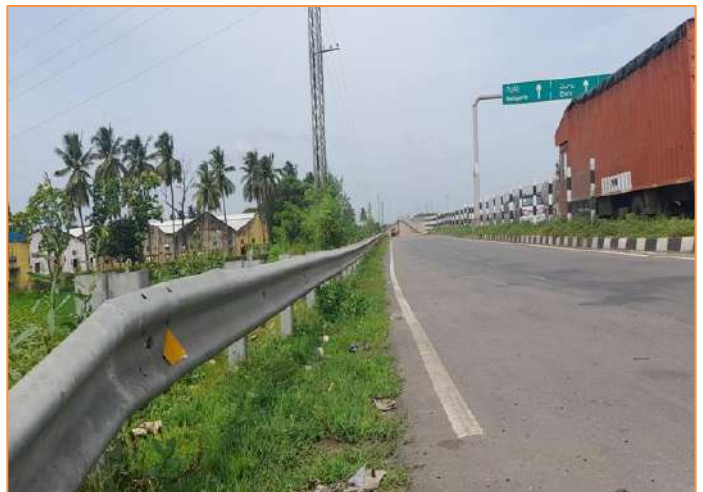
W beam Crash Barrier at km. 85+204
