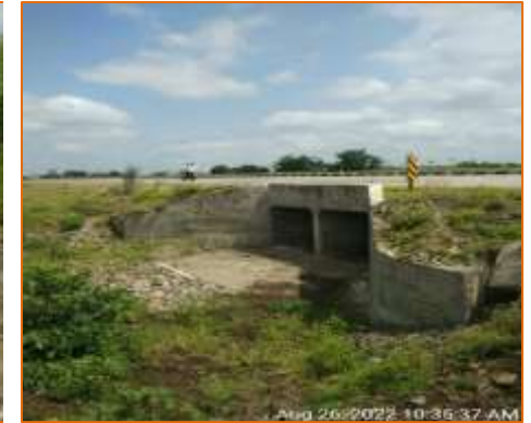
Box culvert at km. 126.643 - LHS (Reconstruction)
