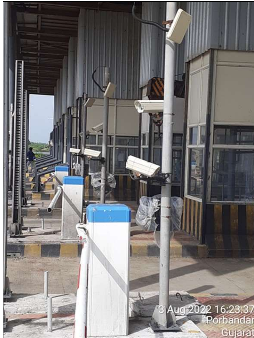
Figure 9-3 RFID ETC Reader mounted on Pole
