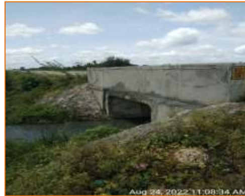
Box culvert at km. 101.823 - RHS (New Construction)
