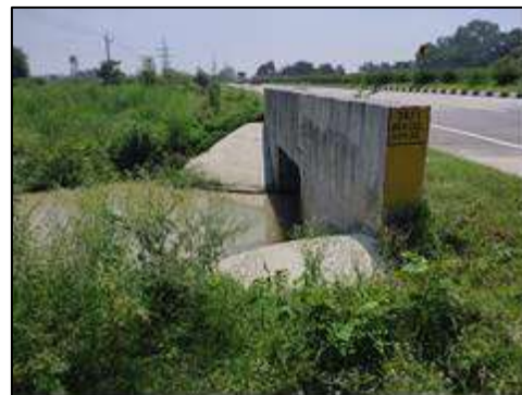
Box Culvert at km. 37+480
