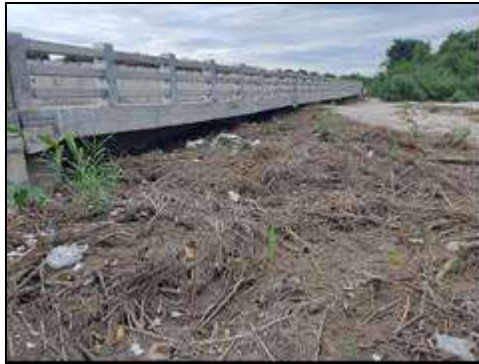
Minor Bridge at km. 72+134 opening blocked (Structure View)
