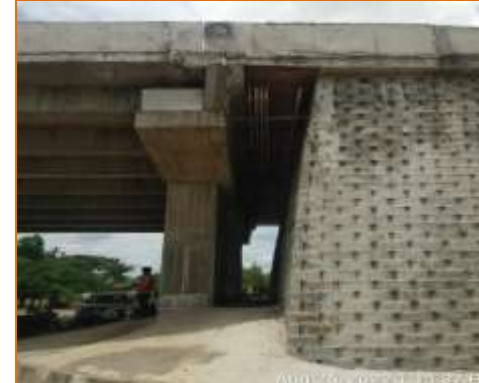
De-shuttering at bottom @ A1 & A2 Side of Flyover at km. 117.935 (RHS)
