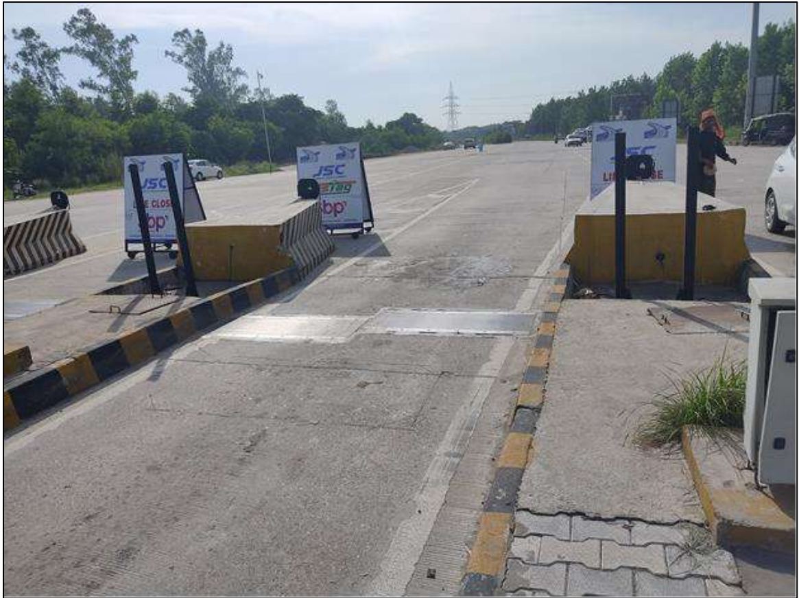
Figure 9-12 Medium Speed Weigh in Motion (MSWIM)
