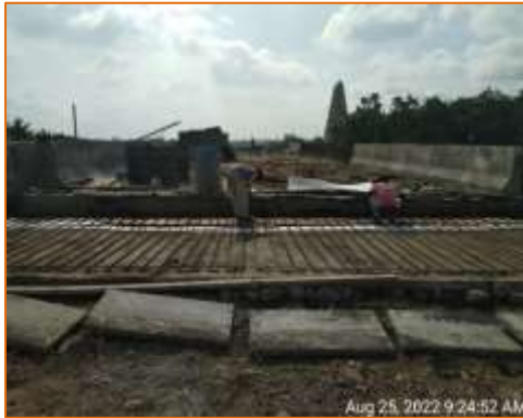
Approach slab work @ A2 side of Flyover is in progress at km. 136.857 (LHS)
