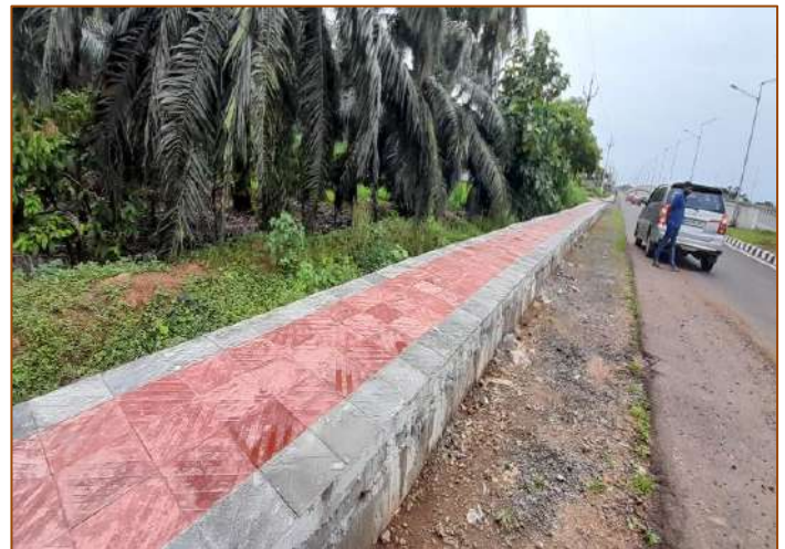
Built-up Drain cum footpath at km. 36+450
