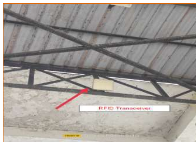
Figure 9-2 RFID Transceiver
