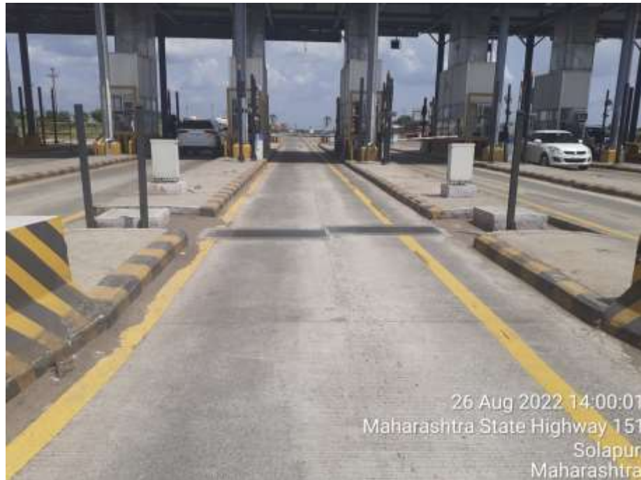
Figure 9-7 Medium Speed Weigh in Motion
