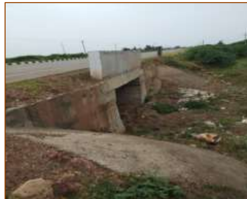
Slab culvert at km. 444+062 (RHS)
