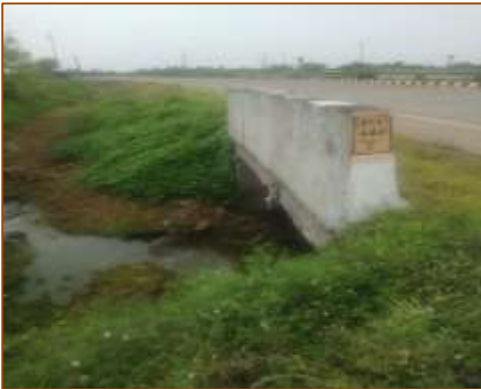
Slab culvert at km. 439+458 (LHS)
