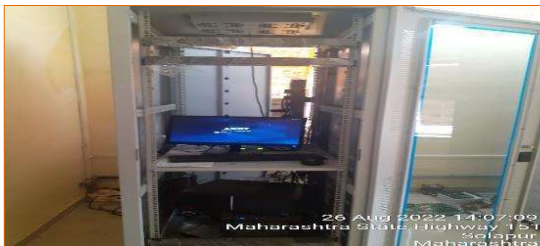
Figure 9-8 Medium Control Room Equipment – Server & Switch rack
