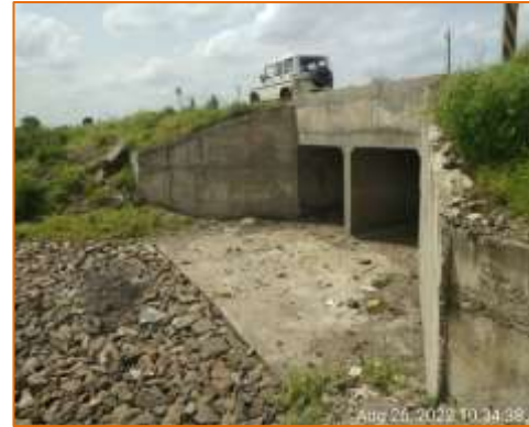
Box culvert at km. 126.643 - RHS (Reconstruction)
