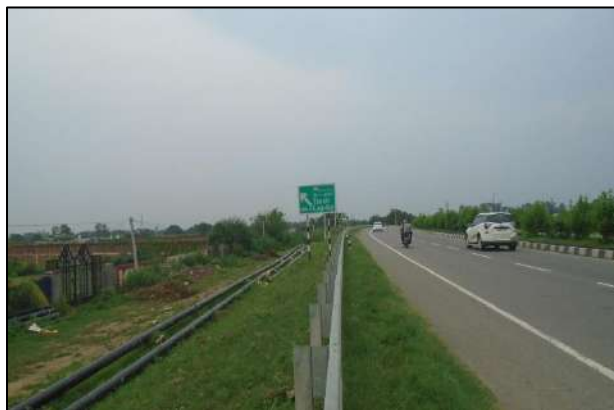
Crash Barrier at high embankment
