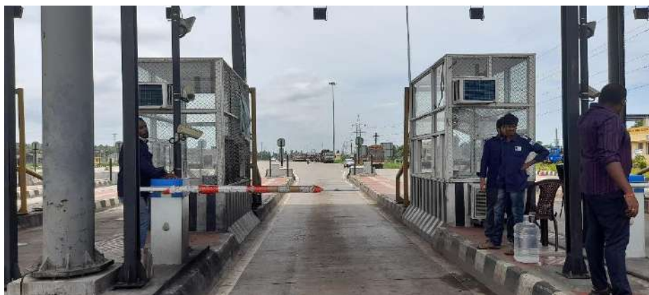
Figure 9-6 Automatic Lane Barrier
