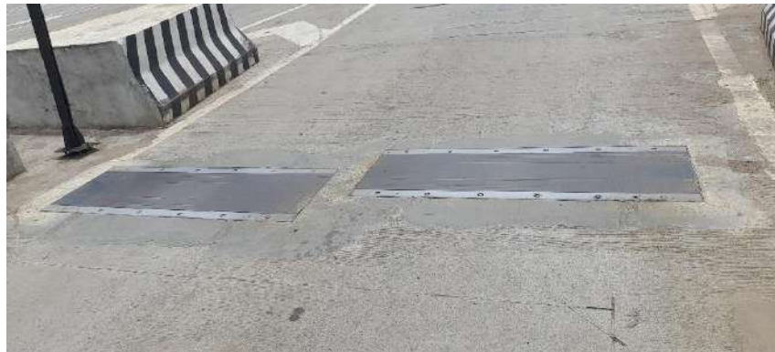
Figure 9-11 Medium Speed Weigh in Motion (MSWIM)
