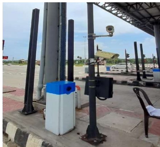
Figure 9-8 LPIC and AVC Cameras
