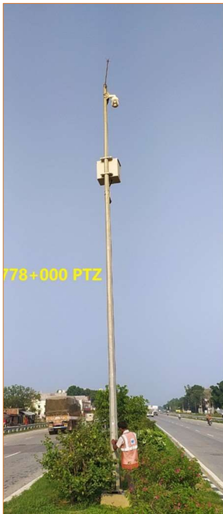
Figure 9-9 PTZ camera at km. 778.000
