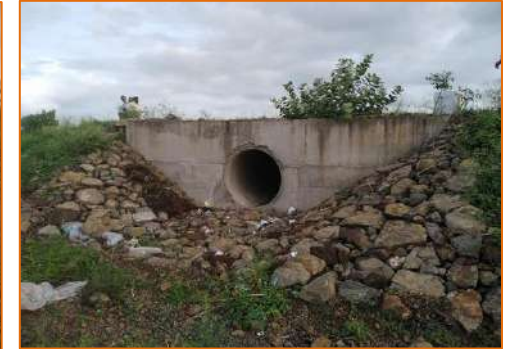
Pipe culvert at km. 310+423
