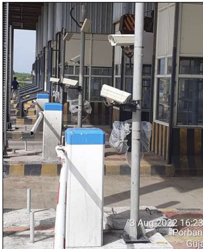
Figure 9-8 LPIC and AVC cameras
