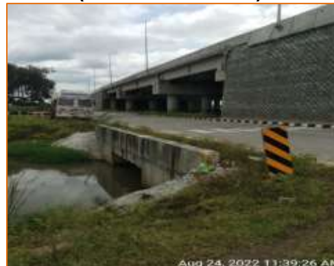
Box culvert at km. 103.850 - RHS (MCW & SR - New Construction)
