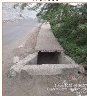
Built-up drain from km. 400+319 to km. 400+700 (LHS)
