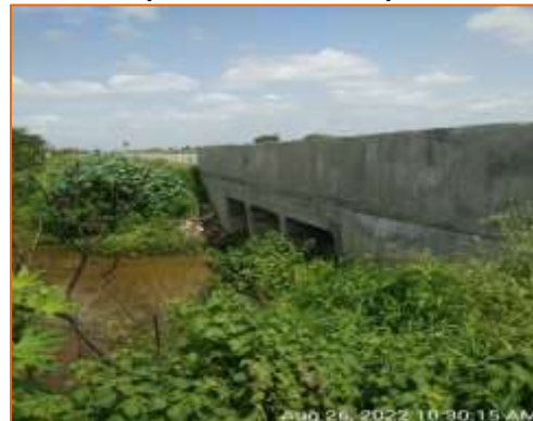
Box culvert at km. 128.229 - LHS (Reconstruction)
