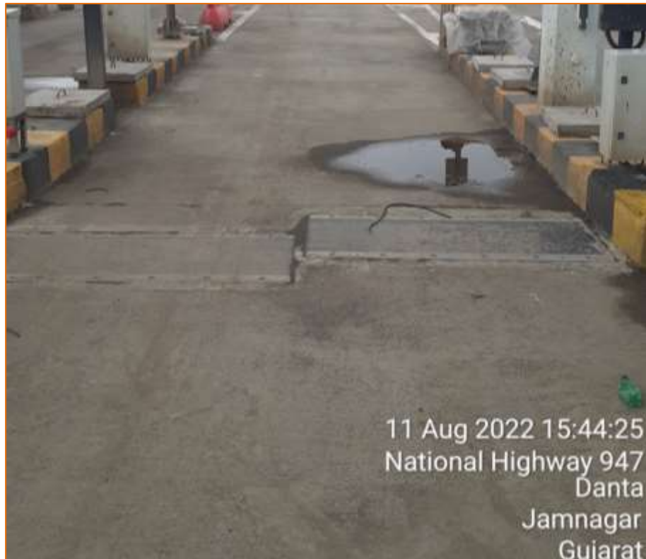
Figure 8-7 Medium Speed Weigh in Motion (MSWIM)
