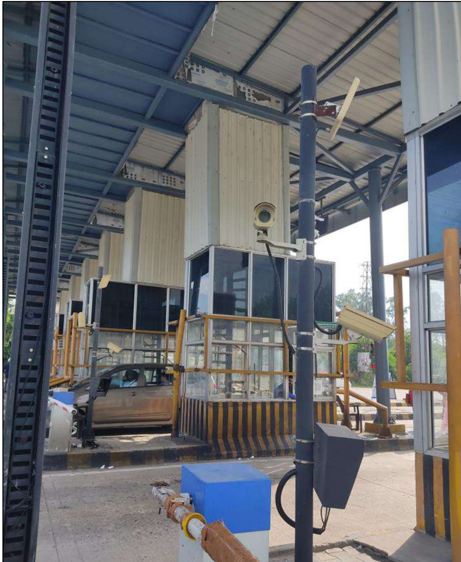
Figure 9-9 LPIC and AVC Cameras
