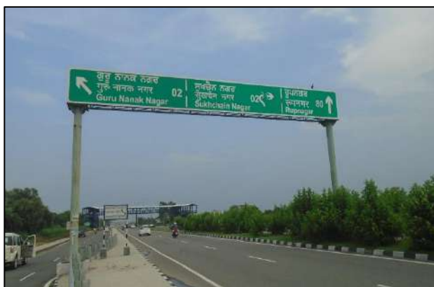
Overhead Gantry Sign Board at km. 8+400
