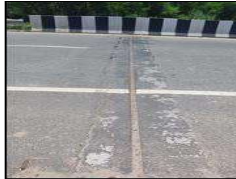
Minor Bridge at km 59+237 (Expansion Joint)
