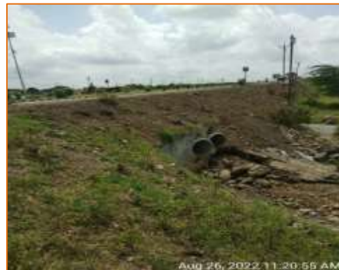
Pipe Culvert at km. 117.423 - LHS (Widening)
