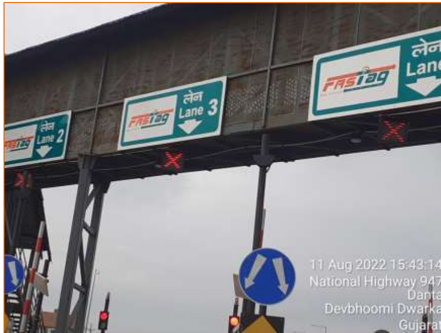
Figure 8-5 Over Head Lane Signal (OHLS)
