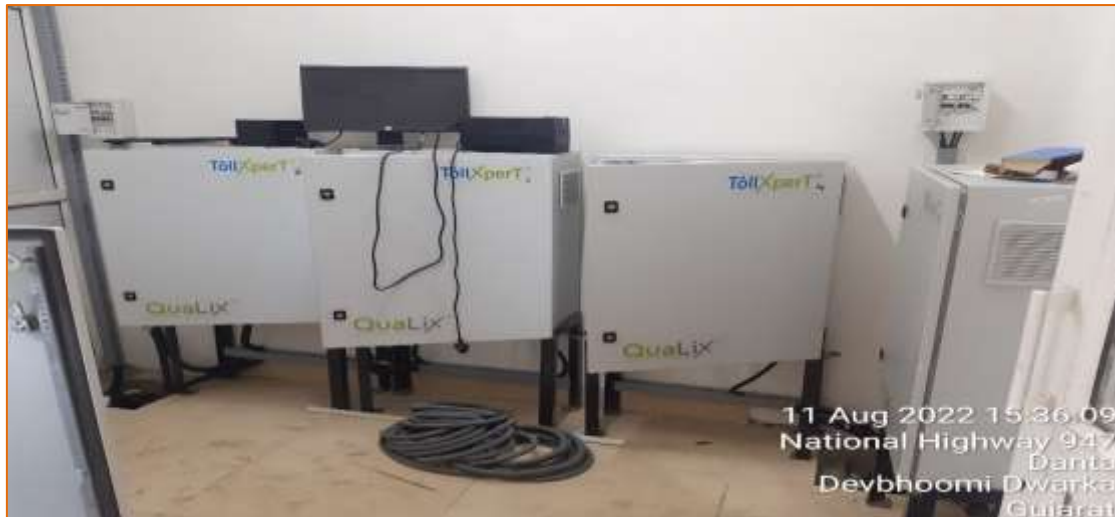
Figure 8-3 Lane Controllers for normal ETC lanes
