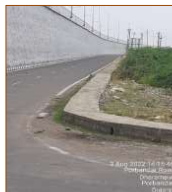
Built-up drain from km. 390+170 to km. 390+953 (LHS)
