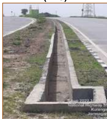
Median longitudinal drain from km. 472+000 to km. 473+000
