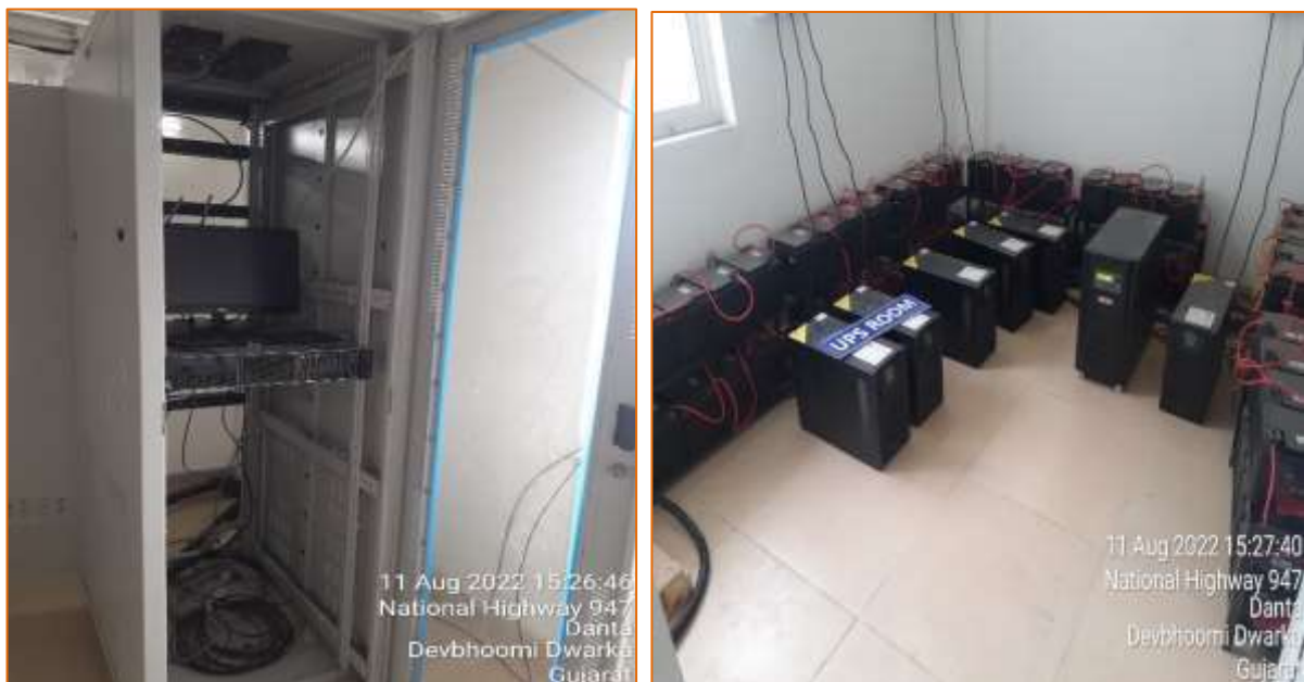
Figure 8-8 Control Room Equipment - Server & Switch rack/UPS Room
