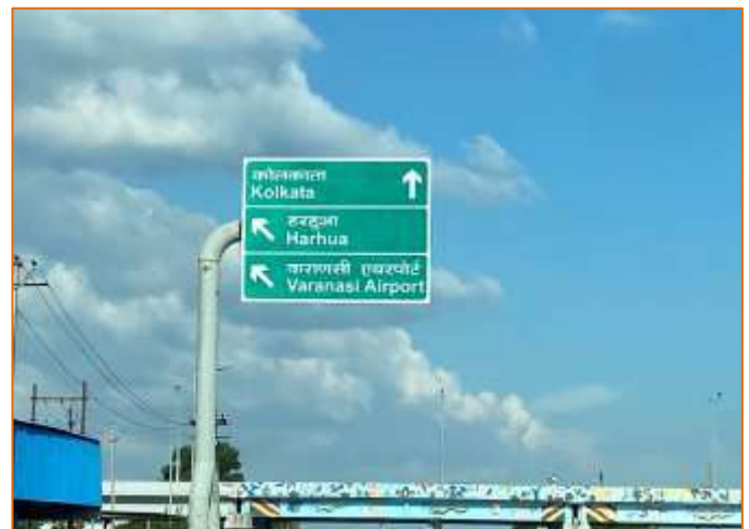
Cantilever Gantry Sign at km. 782+500
