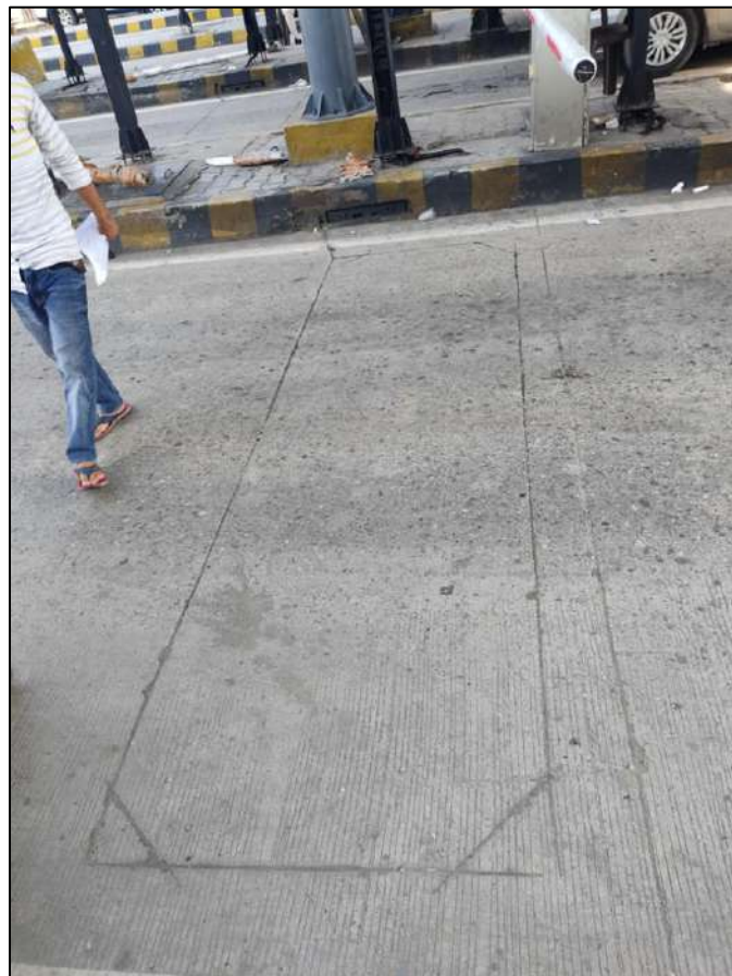
Figure 9-6 Inductive loop
